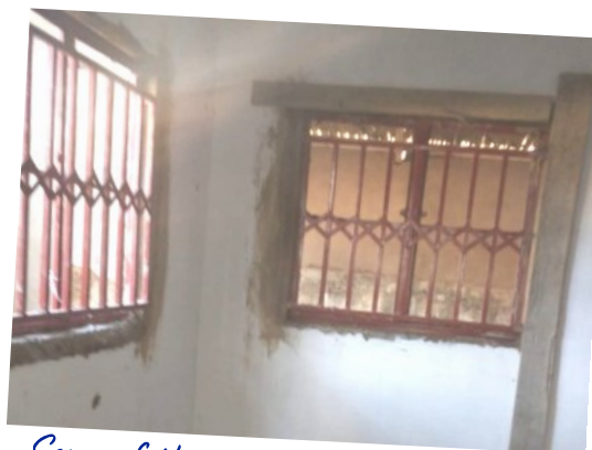
Some of the newly installed windows at Domingos' church
