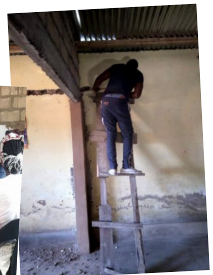
The electrician is making a start already
