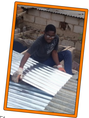
The new roof taking shape
