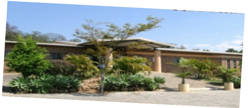
The front of the Nelspruit Calvary Church building
